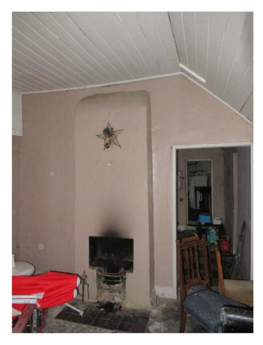
Plate No. 11. General internal view showing the chimney breast in the east room in the cottage. Note the timber-sheeted ceiling, with the collar ties raised above the wall heads.
